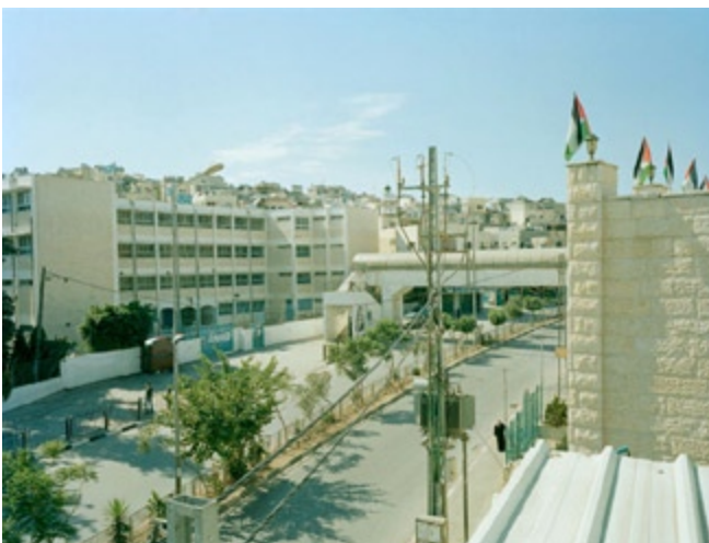
The bridge from Dheisheh Refugee Camp to Doha City. The only bridge built by Palestinians in Area C, it connects the camp to the entirely new, refugee-inhabited municipality of Doha. Not only the physical link between the camp and its expansion, the bridge also marks the absolute centrality of the camp for the refugee community living beyond its borders. – photo: Lisa Bergmann / Karlsruhe University of Arts and Design (HFG) for Campus in Camps, 2011
