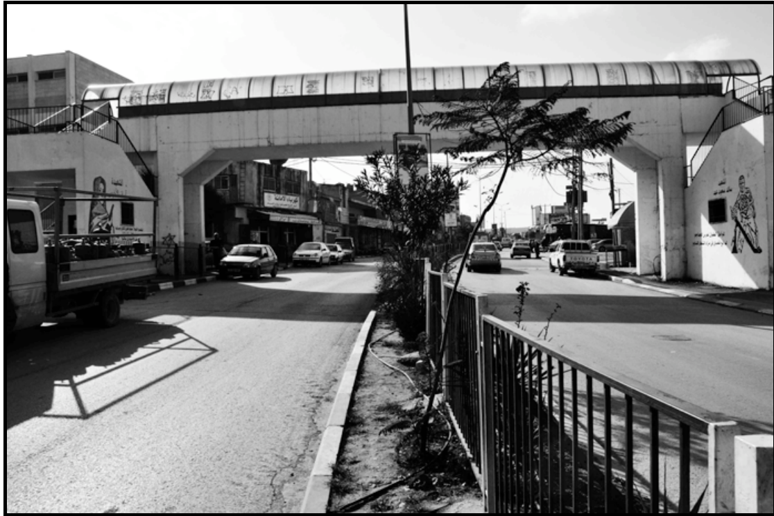
Figure 1 - Pedestrian bridge linking Deheishe and Doha [Photograph N. Abourahme]
