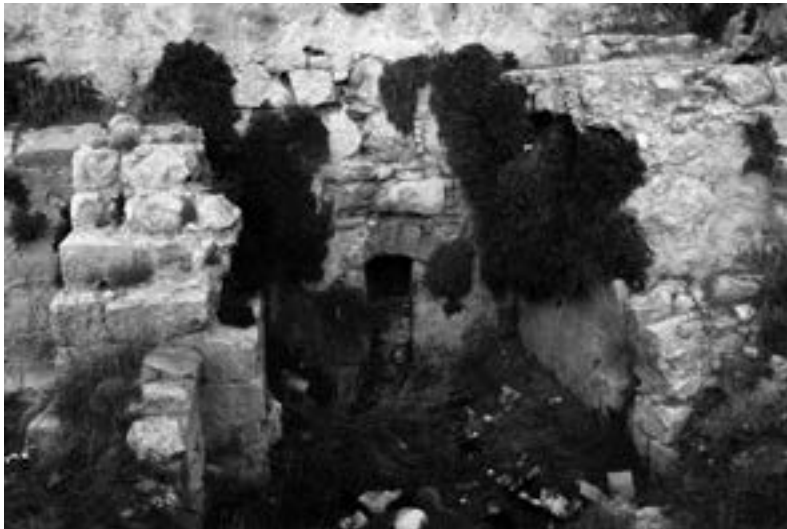
The Ancient Roman pool in Arroub and the beginning of the aqueduct.
